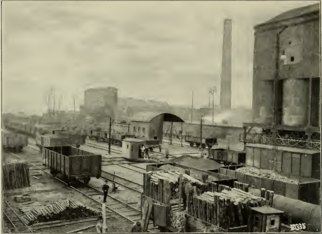
FIG. 11. SURFACE PLANT LIGHTED BY ARC LAMPS.
